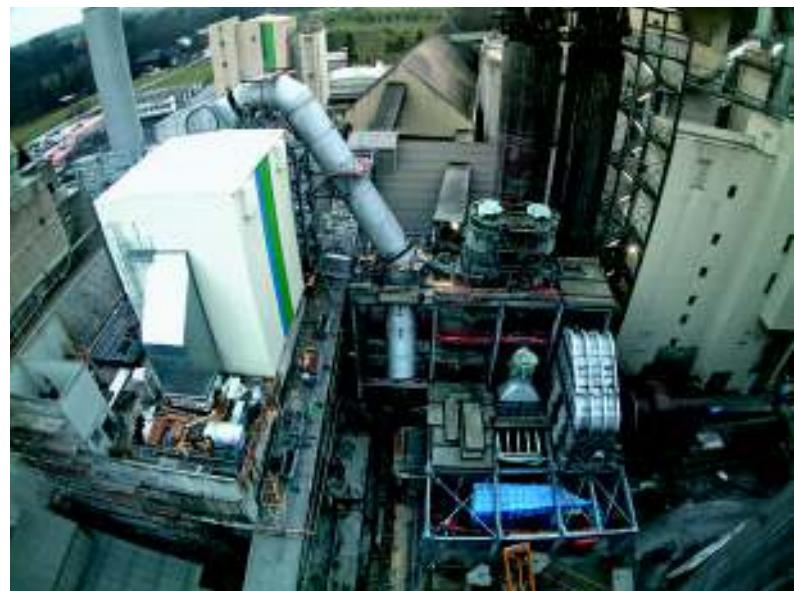
**13 The clinker cooler has been hoisted in and the kiln hood is mounted**
