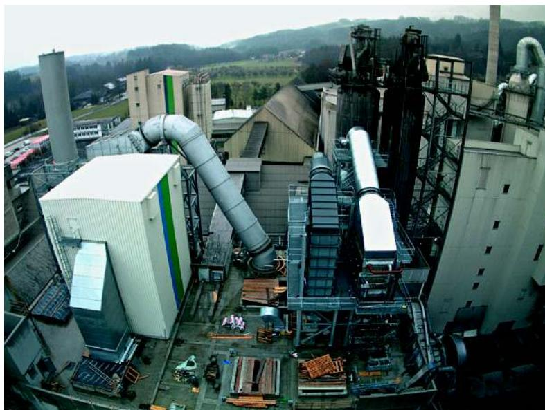
**14** The heat exchangers for the heat recuperation from the mid-air are mounted
